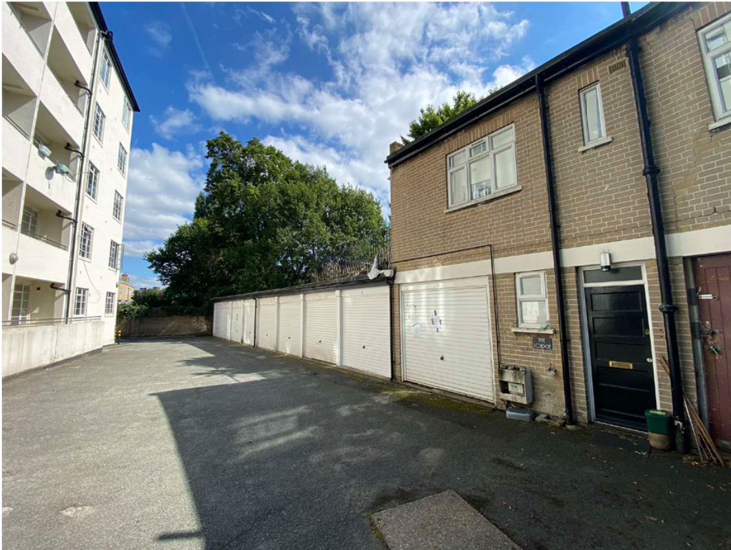
Garage block to the rear of the site
