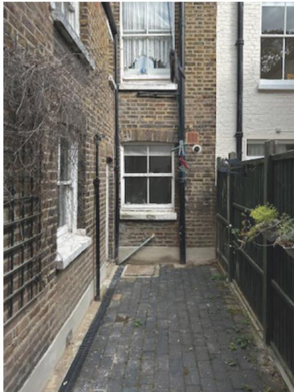
Figure 3 Rear elevation of application site (Source: submitted documents)
