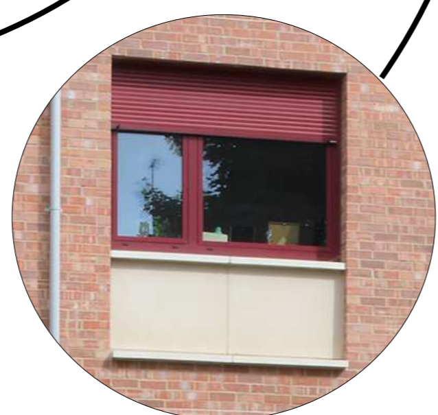
External solar shading to reduce overheating of homes
